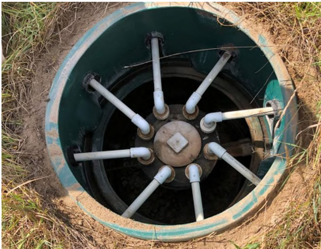
Figure 17: View of the 1-to-8 way distribution valve. The valve receives effluent from PC1 via a pressurized forcemain entering from below and discharges to the Ecoflo treatment units.
