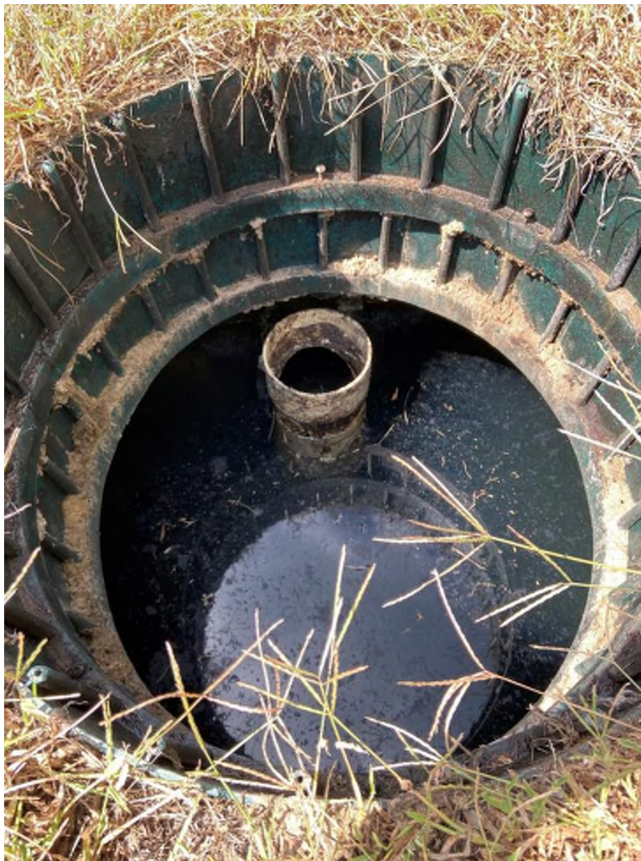
Figure 2: Inlet chamber of ST1. The inlet baffle was present and in good condition. The fluid level was elevated as the pumps in the tank adjacent were not operational.
