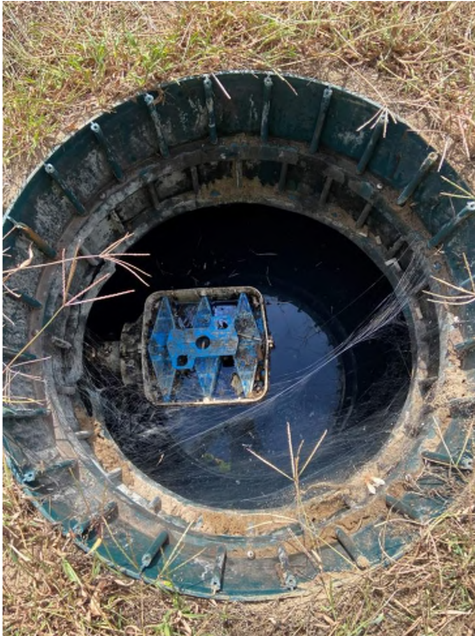
Figure 3: Outlet chamber of ST1. The outlet pipe was equipped with a commercial grade effluent filter. The filter was relatively clean and in good operational order.
