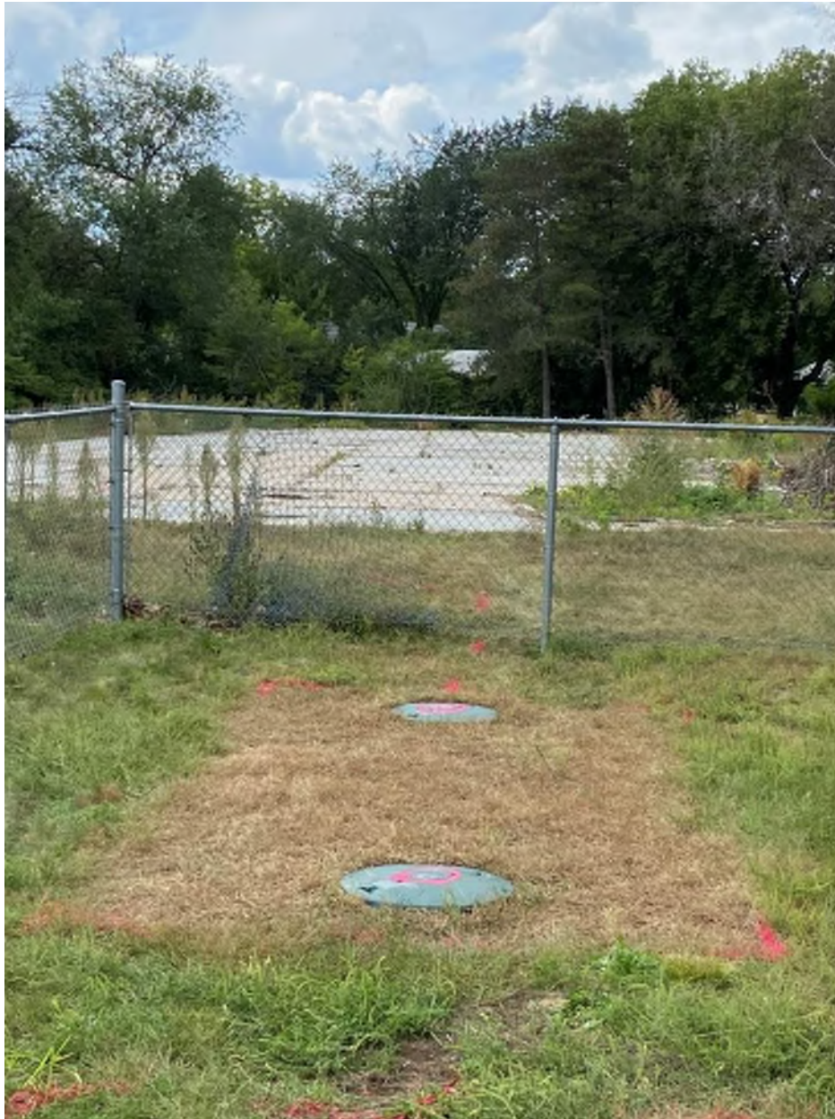
Figure 1: Location of Septic Tank 1 (ST1). The 150 mm diameter sewer pipe is identified with paint markings visible in the background of the photo.
