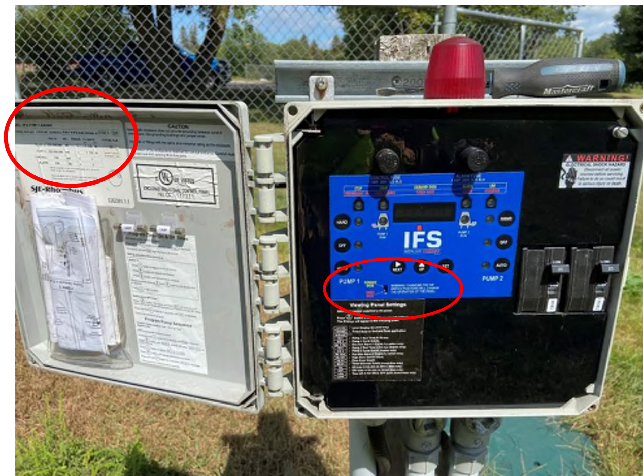
Figure 10: The existing pump controller and alarm is an SJE-Rhombus brand IFS series model IFS31W114X8AC. The controller dictates the operation of two (2) sewage pumps which were configured to dose on demand.
