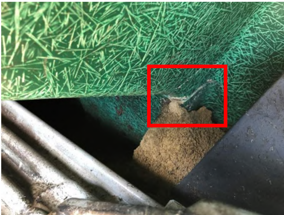
Figure 26: Small 10 cm crack observed in fibreglass shell of Ecoflo #8.
