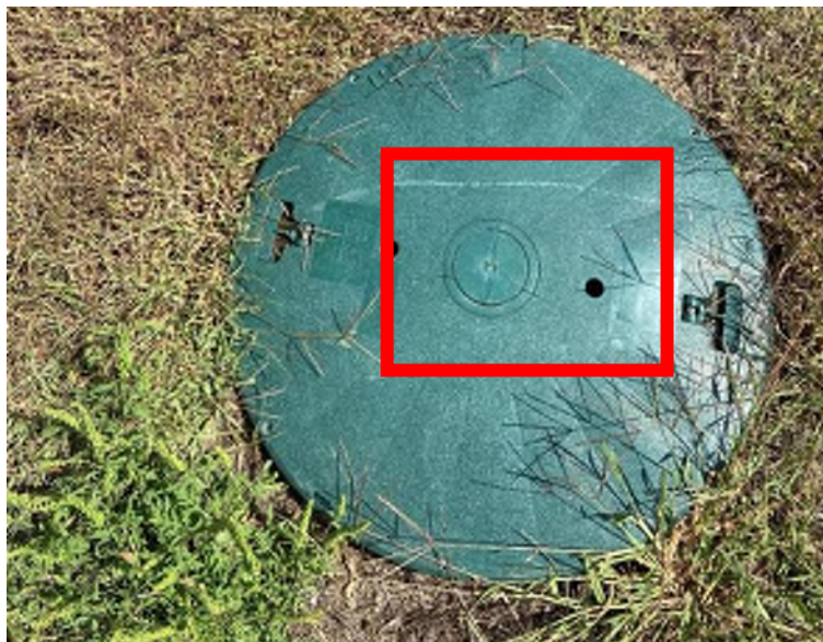
Figure 13: Cracked access lid of PC1.
