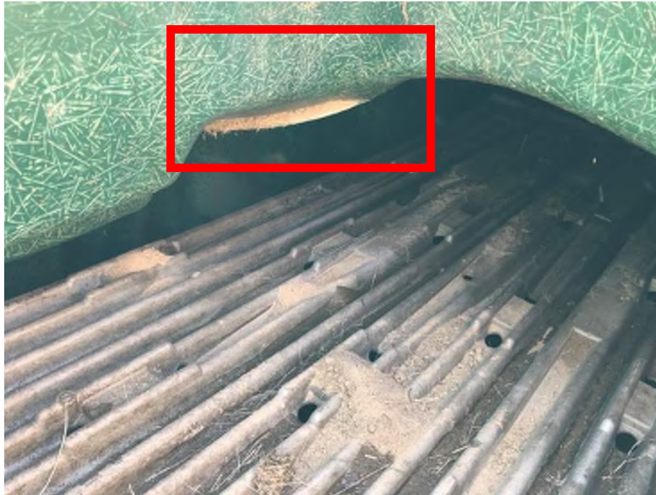
Figure 22: Small 15 cm crack in fibreglass shell of Ecoflo #3.
