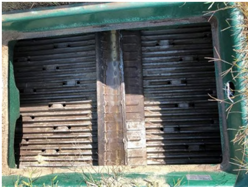
Figure 18: Typical internal view of an Ecoflo ST-650 treatment unit.
