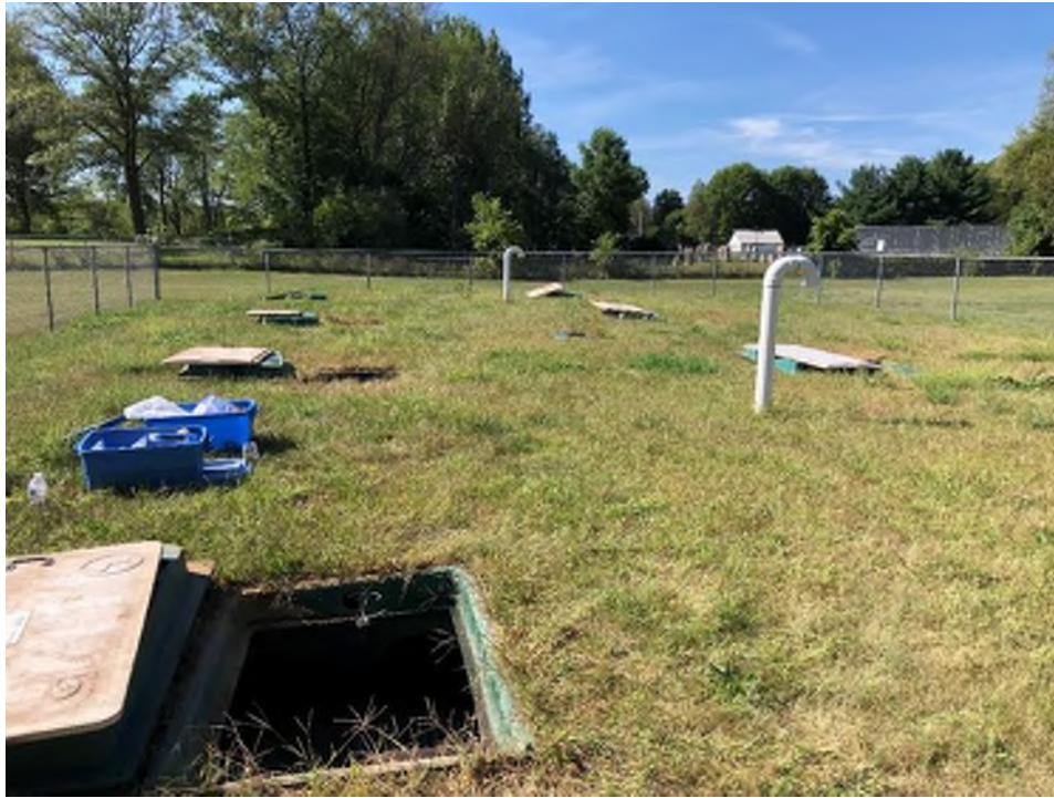
Figure 20: Ecoflo #1 (foreground) appears out of level.
