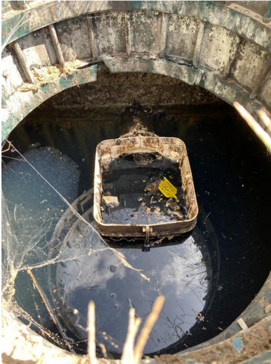
Figure 6: There was plastic garbage floating in the surface scum layer. There was a surface sheen on the top of the fluid in the inlet and outlet chambers of ST1.
