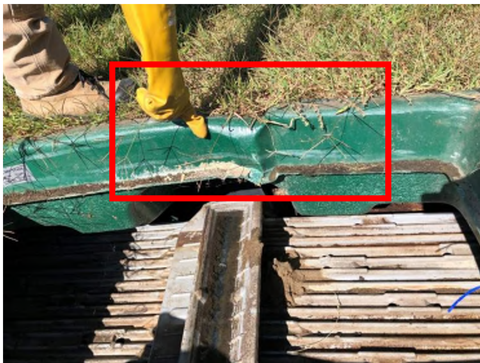
Figure 21: Significant damage to Ecoflo #2 causing difficulties closing lid.
