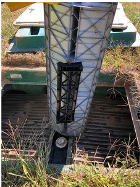
Figure 19: Typical internal view of an Ecoflo ST-650 treatment unit with tipping bucket removed and central port visible.
