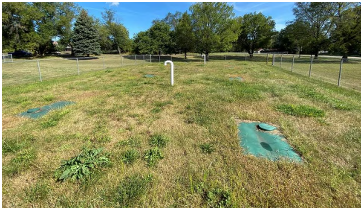
Figure 14: Location of the Ecoflo treatment units and subsurface disposal bed.
