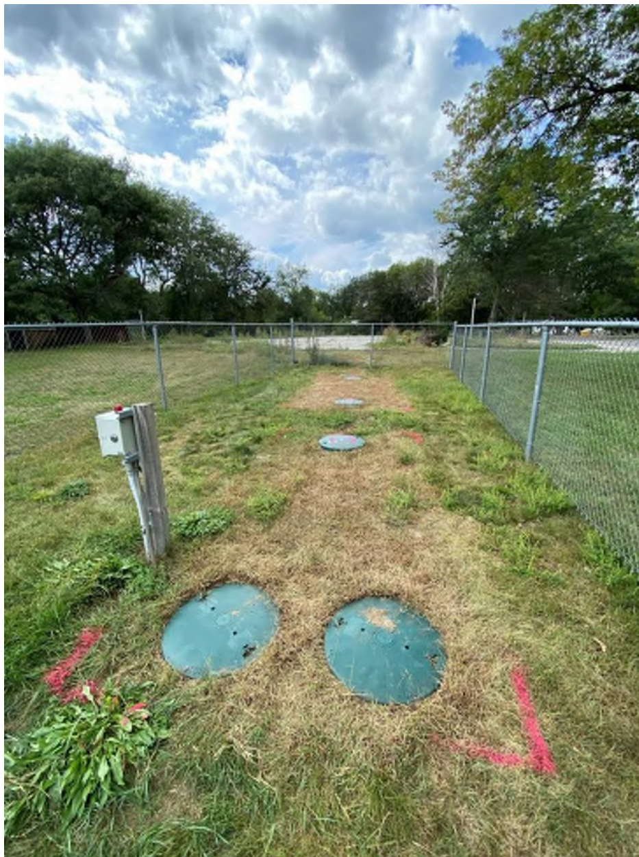
Figure 9: Location of Pump Chamber 1 (PC1) and associated pump controller and alarm system.
