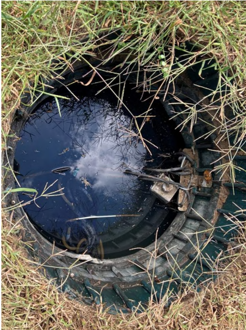
Figure 11: View of PC1 at pump discharge location. As was the case in ST1 the fluid level was elevated as the pumps were not operational. The fluid in the tank may have entered into the grey electrical box.
